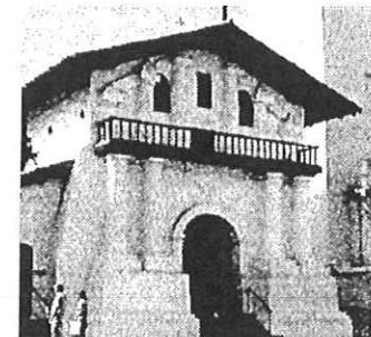
Notice the mausoleum's resemblance to the Mission San Francisco de Asis (Mission Dolores) above. California State Historic Landmark 327
