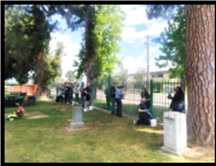
Cleaning and Repainting our wrought iron fence!
