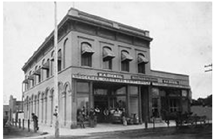
August’s brick office building at 202 W. Center St. (Now Lincoln Ave.) He sold it to his son-in-law, Herman Dickel in 1892.
